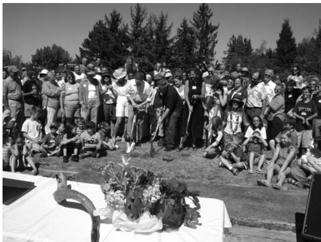
Groundbreaking at Temple Beth Israel.
